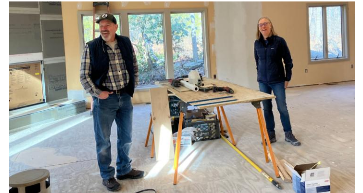
Checking on the renovation project at Camp MH
